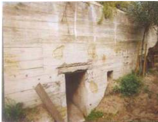
The 502 with walls of 3 m thick. Note the pale yellow colour. (F Philippart)
