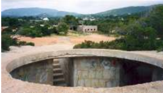
Gun 1 and roof of the tunnel
