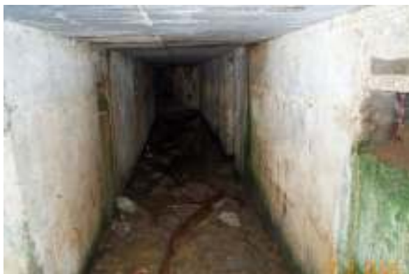
Inside the connecting tunnel.
