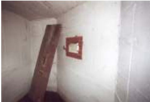
Inside the close defence room.
