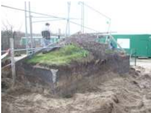
The VF Wasserbunker has quite small dimensions: 5,00 x 2,40 m with 0,50m thick walls
