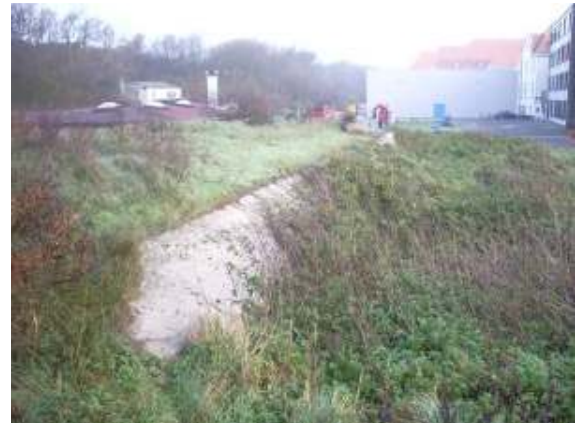
Today, only a small part of the roof is visible. We had to dig to reach inside
