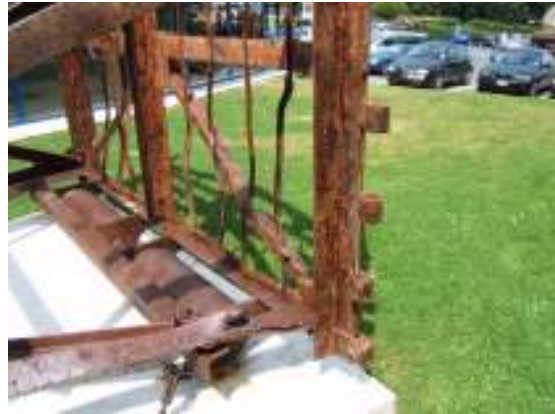
The four hinges on the side of the gate.
