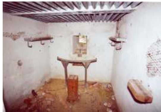
A Chardome mounting inside such a bunker.
