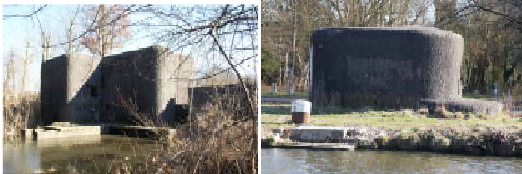
Tapsluis Noord (left) and Tapsluis Zuid (right)
