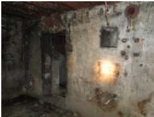
The entrance of the crew room.
