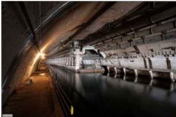
Special dock for repairs.
