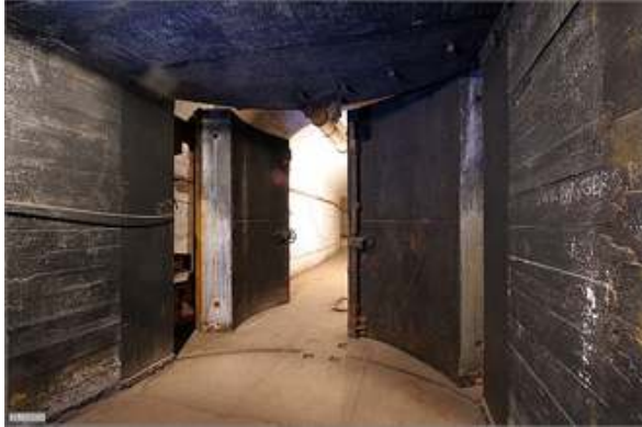
One of the automatic doors.
