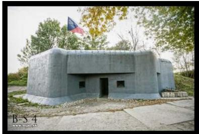
The side exposed to the enemy is completely covered by earth, the weapons being installed to cover the intervals between the bunkers. The main armament was in this case one Czechoslovakian built 47mm antitank ŠKODA oun that was state of the art at the time. It could penetrate 5 cm of armor and therefore knock out the panzers of the period at a range of more than1000m.
