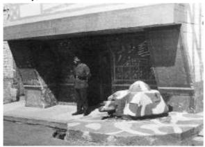
The bunker is a Vf construction and a Sonderkonstruktion (special construction). It has a crew room that connects to a corridor with two entrances and there's another entrance on the street side. The roof of the bunker is a combat position for individual weapons and machine guns.
