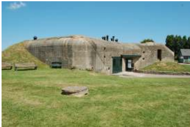
The Regelbau 611 is by far the largest combat casemate of the Merville battery.
