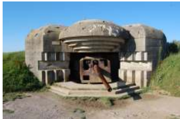
Front view of one of the four combat bunkers with clearly visible the openings to give the gun some more range in both directions.
