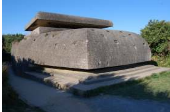
Front view of the fire control bunker
