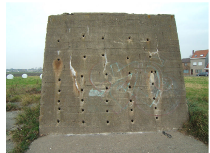
The drilling holes in the concrete blocks.
